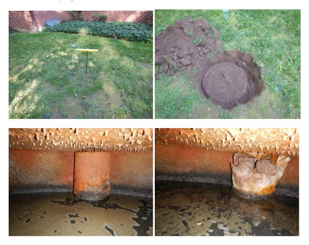
Water was run into the tank from the home. During the running of the water, the level remained constant, exiting the tank, out into the absorption area, with no issues. All internal waste, water lines were verified to be entering the septic tank.
