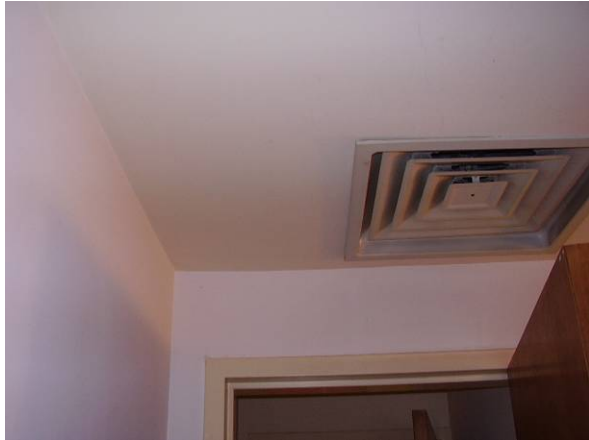
Photo #7 View of plaster wall and plaster ceiling.
