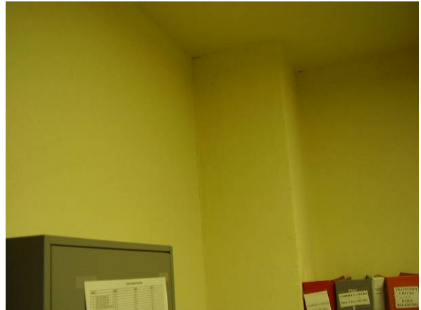
Photo #10 View of texture covering concrete brick wall.
