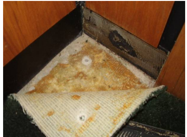
Photo #4 View of yellow carpet mastic and brown cove base mastic.
