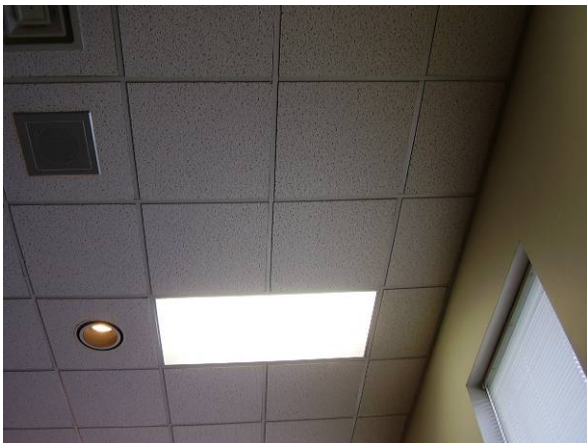
Photo #5 View of 2'x2', suspended ceiling tiles, white, pinhole, small cut, recessed.
