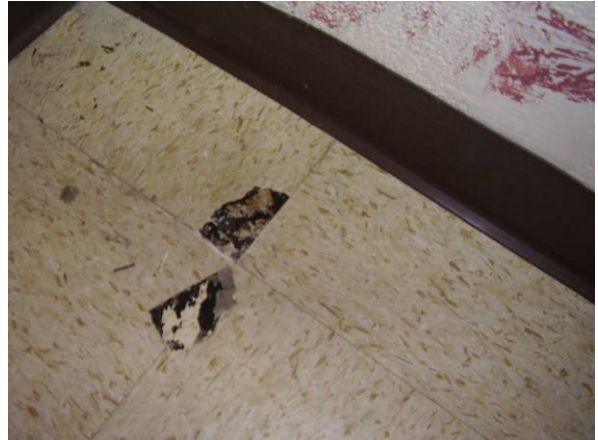
Photo #8 The 12"x12", vinyl floor tile, off white with green specks and black mastic is considered an ACM.
