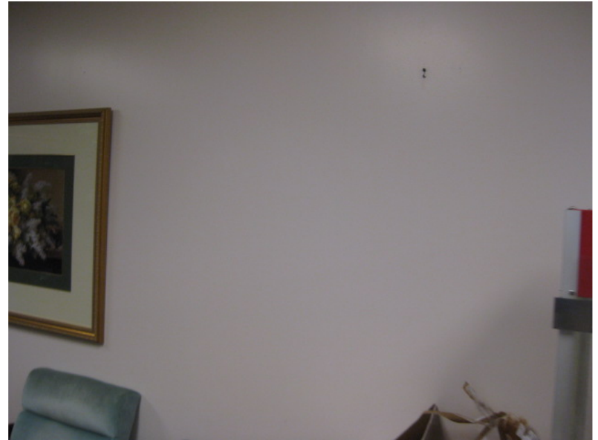
Photo 10: View of drywall located throughout exterior walls.
