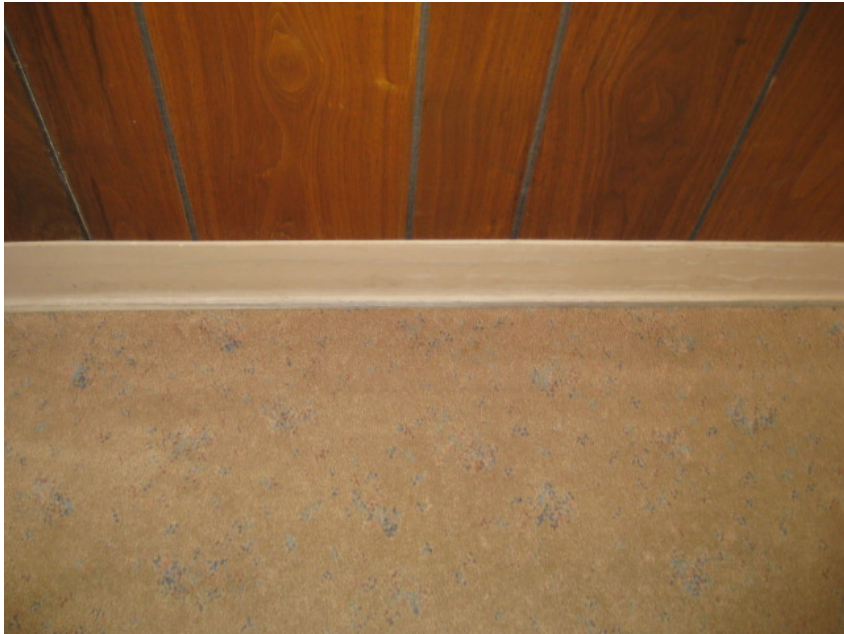
Photo 9: View of 4" cream basecoat associated w/mastic located in the west offices.
