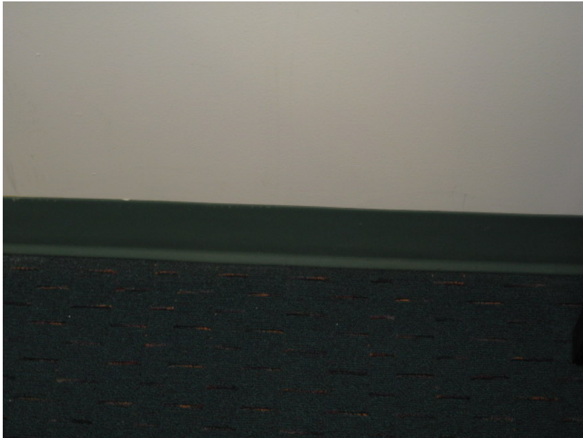
Photo 5: View of 4" teal basecove associated w/mastic located throughout offices
