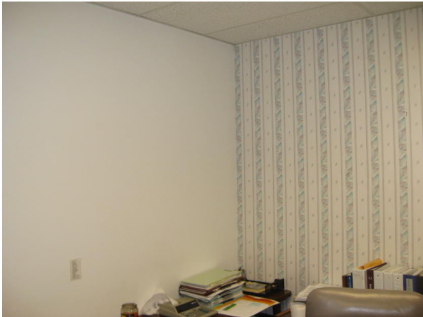
Photo 11: View of drywall located throughout interior demising walls.
