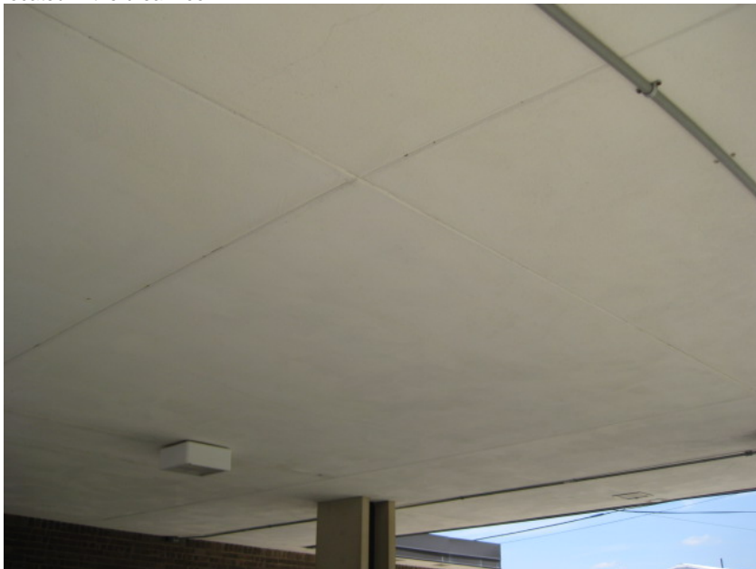
Photo 15: View of concrete ceiling under drive-thru.
