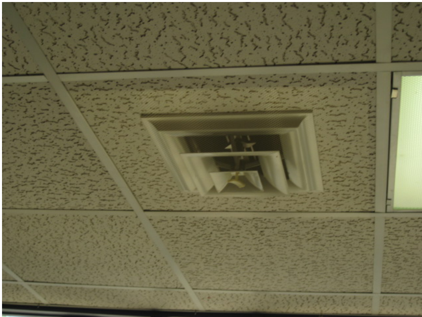
Photo 7: View of 2' x 2' white ceiling tile w/fissures located in the entrance of bank.
