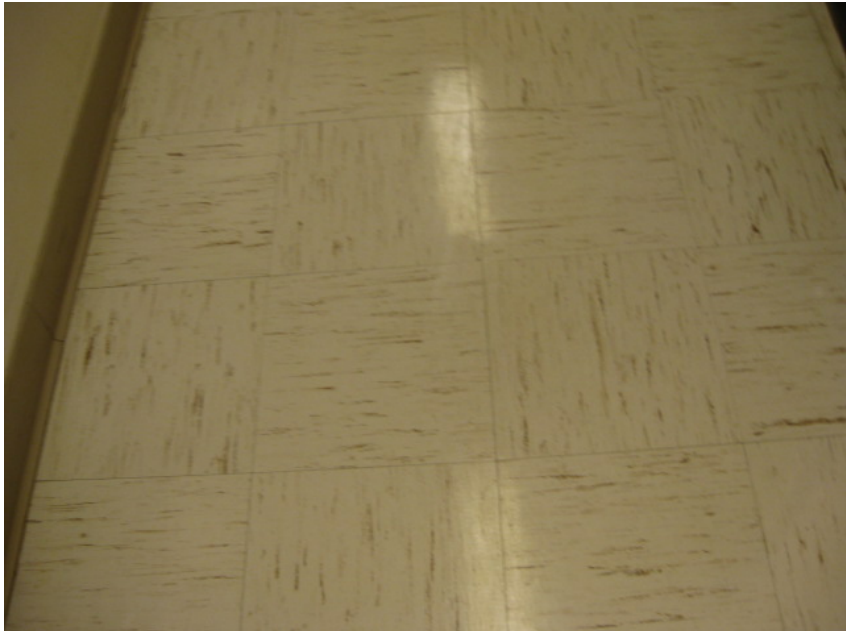
Photo 13: View of 12" x 12" white floor tile w/brown streaks associated w/mastic located in the break room.
