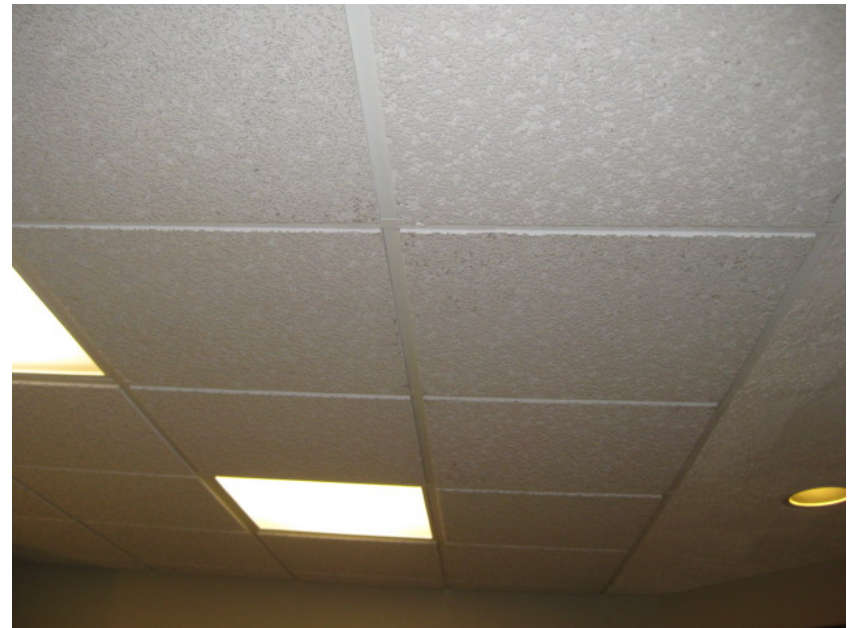
Photo 8: View of 2' x 2' white ceiling tile w/rough surface located in the side entrance .
