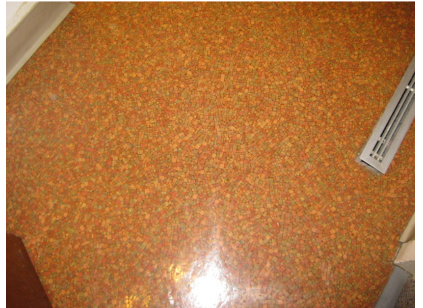
Photo 12: View of ACM brown linoleum associated w/ACM mastic located throughout men's and women's bathrooms.
