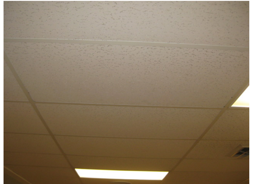
Photo 4: View of 2' x 4' white ceiling tile w/fissures located throughout offices.
