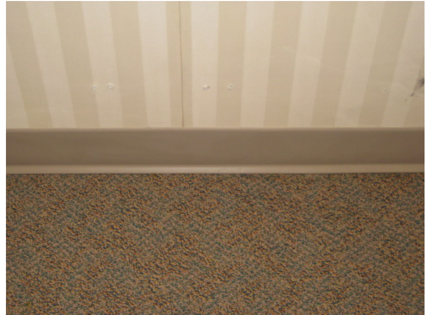
Photo 6: View of 4" tan basecove associated w/mastic located in the break room.
