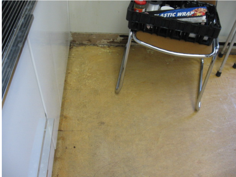
Photo #1 HA01, 021 – 12" x 12" Floor tile, green and white mottled and associated mastic
