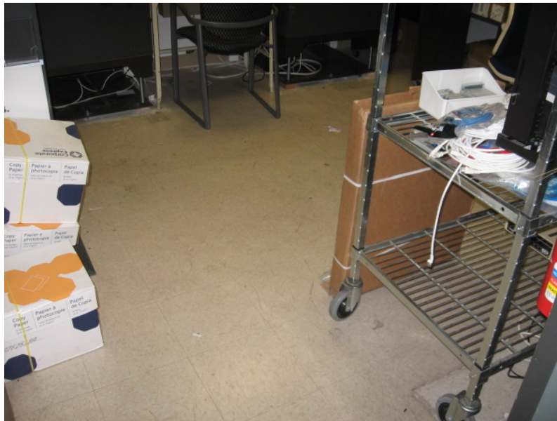
Photo #6 HA 08, 09 – 12" x 12" Floor tile, tan with beige spec and associated mastic
