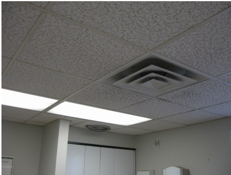
Photo #2 HA 03 – 2' x 2' Lay-in ceiling tile
