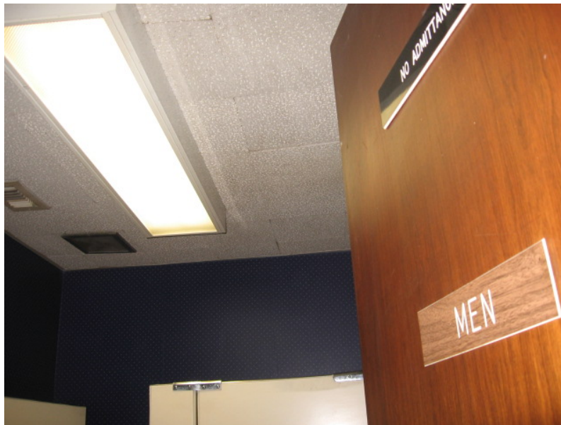
Photo #3 HA 04 – 1' x 1' spline ceiling tile
