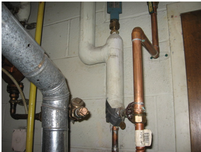
Photo #4 HA 05 – TSI Domestic pipe fitting insulation
