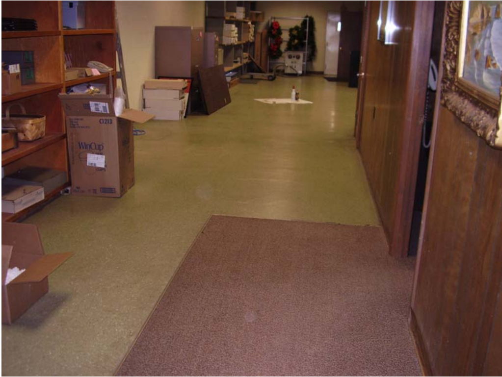
Green Floor Tile in Storage Room
