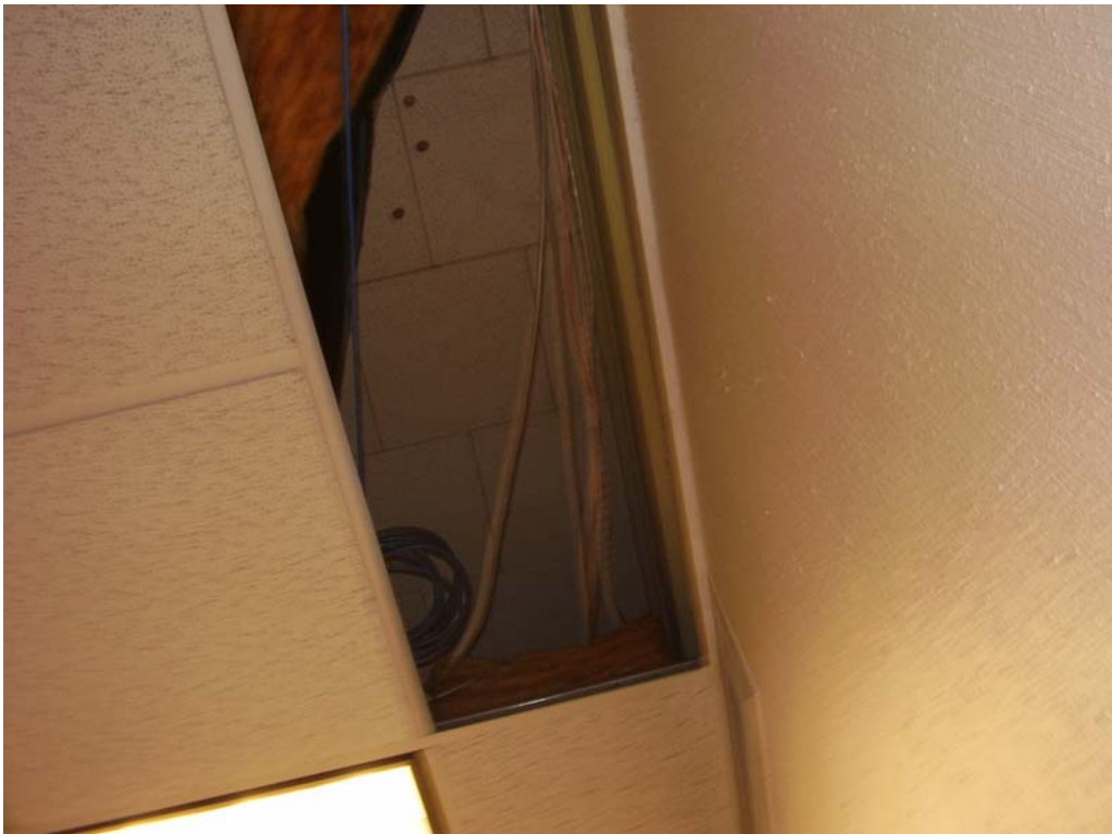
Ceiling Tile above Ceiling Tile in Lobby
