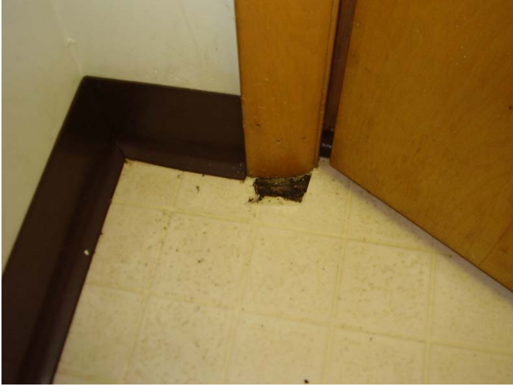
Floor Tile and Mastic under Sheet Flooring
