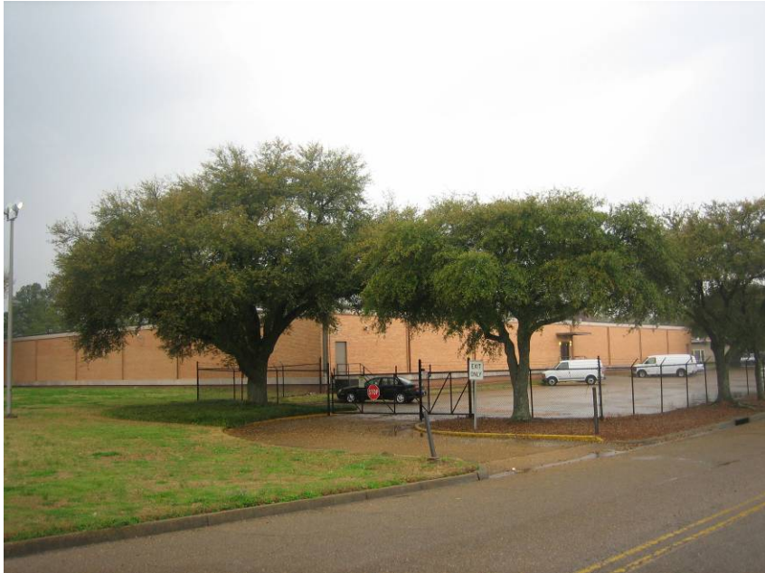
Photo 1: Exterior of building
