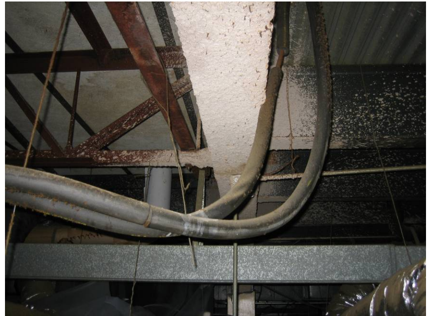
Photo 4: Asbestos-containing fireproofing above the kitchen.
