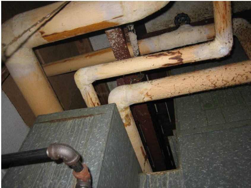
Photo 3: Asbestos-containing hard pipe elbows above the kitchen.
