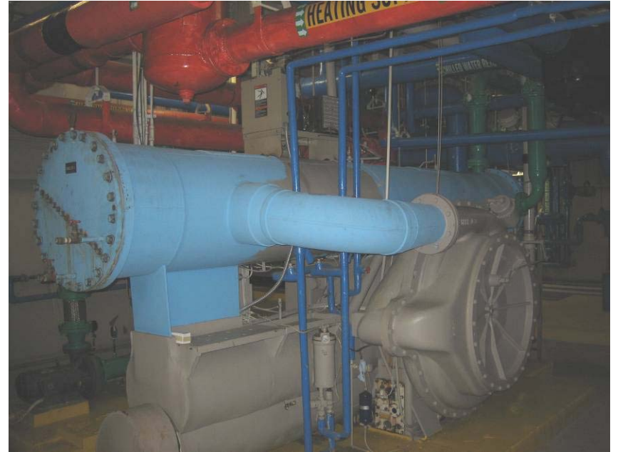
Photo 6: Chiller unit in the mechanical room.
