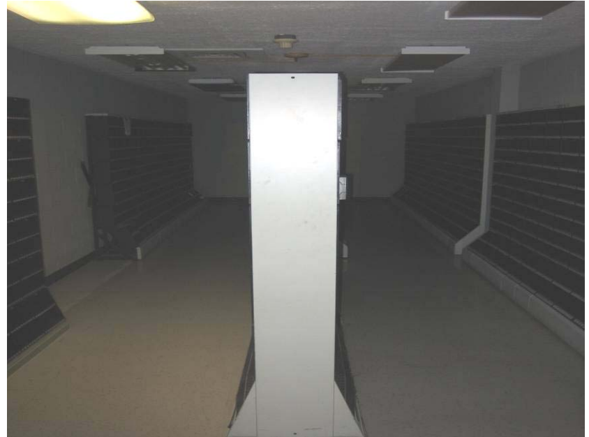
Photo 2: Vacant tape vault, asbestos-containing floor tile and ceiling texture is in this room.
