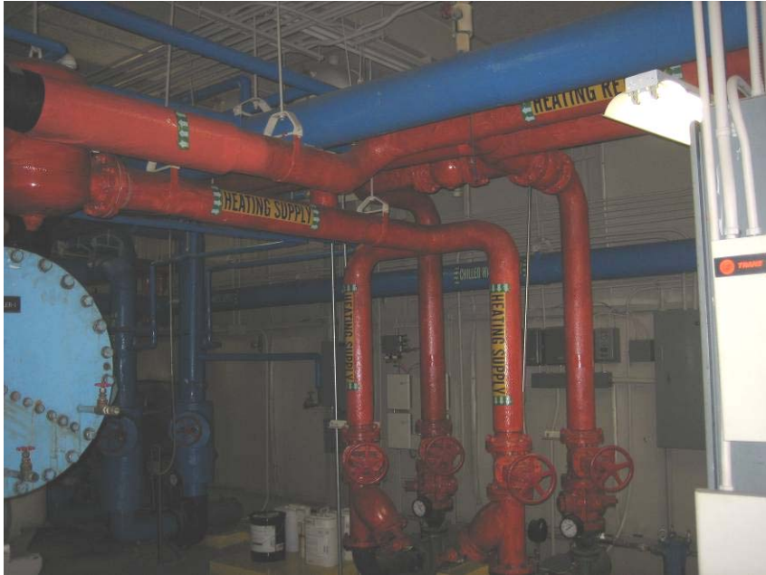
Photo 5: Asbestos-containing pipe elbows in the mechanical room.
