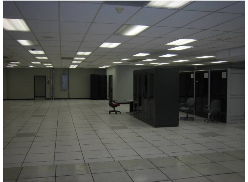
Photo 12: Overview of server room.
