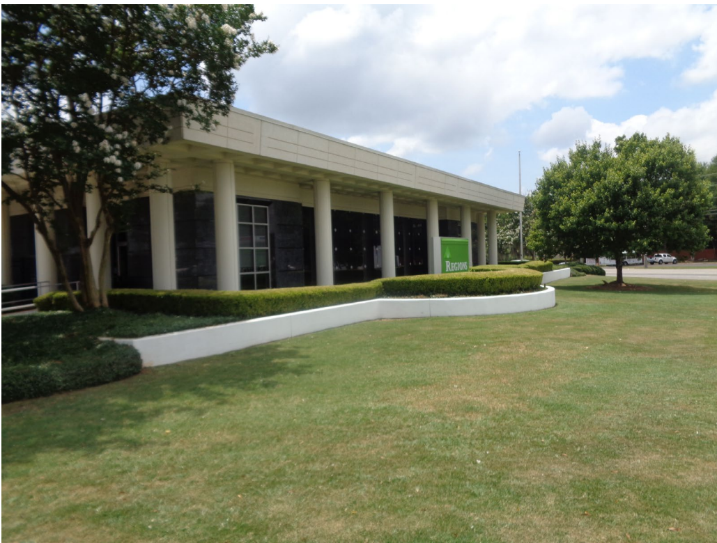
Photo No. 1: Front view of the subject property.
