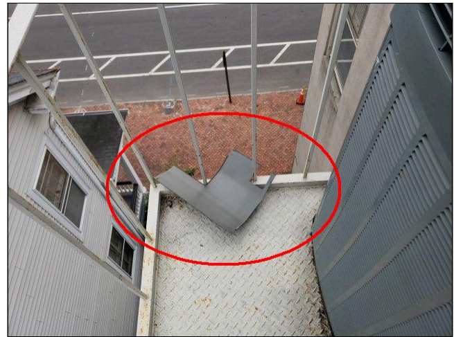
9.1 OUTDOOR/CONDENSING UNIT(S) Photo 7
