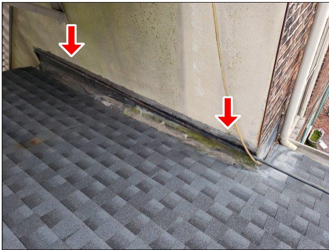
1.5 EXPOSED FLASHING Photo 1
