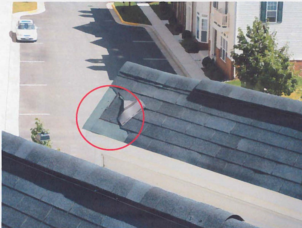
Photograph 5 – Wind damaged shingles.
