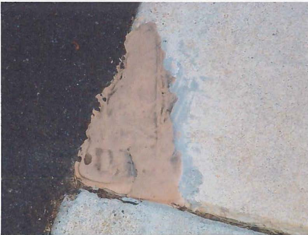
Photograph 12 – Substandard/unsightly repair at concrete sidewalk.
