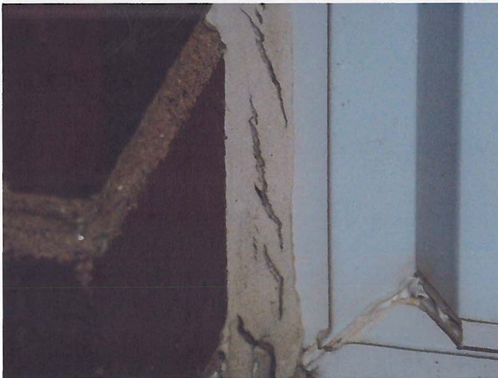
Photograph 2 – Torn sealant.
