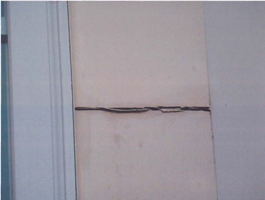
Photograph 3 - Debonded sealant.
