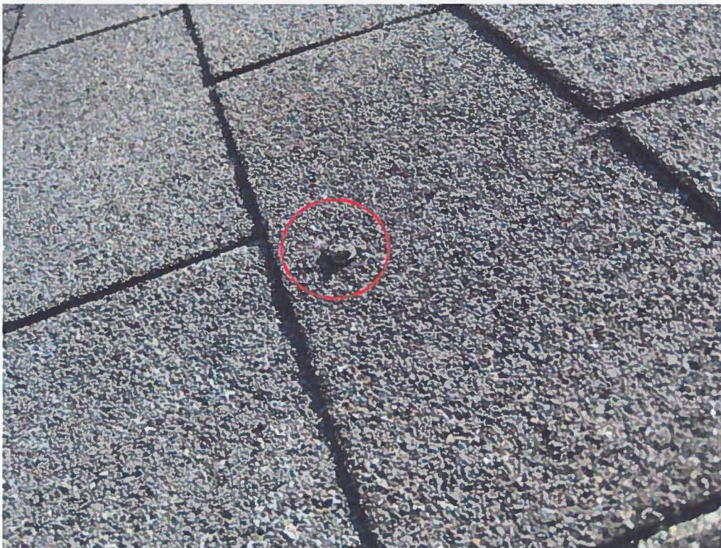
Photograph 4 - Face-nailed shingle.
