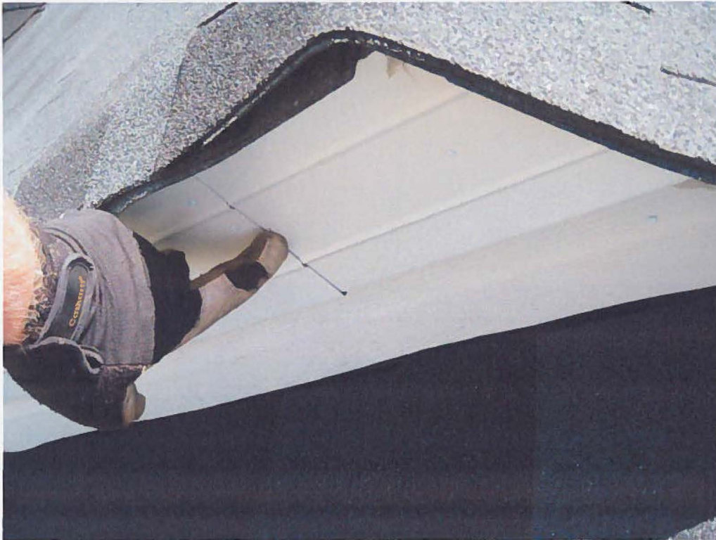
Photograph 1 – Improperly lapped trim cladding.
