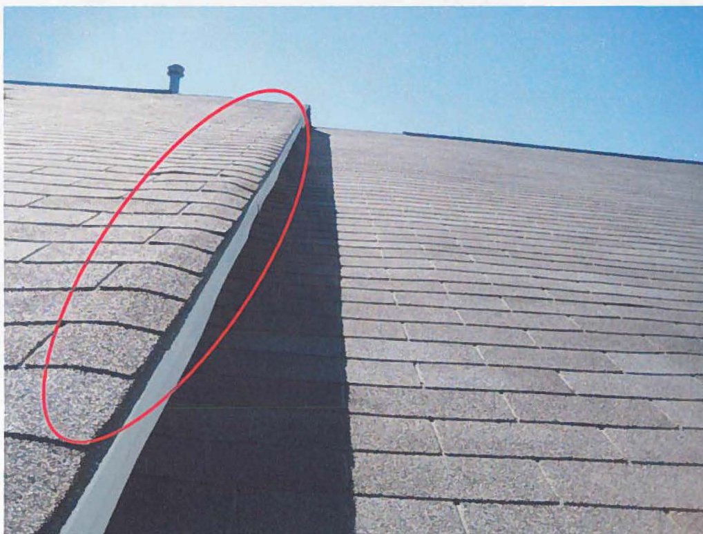
Photograph 6 – Shingles distorted due to excessive overhang.
