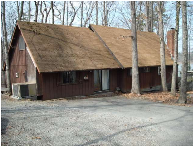
Main Structure Photo
