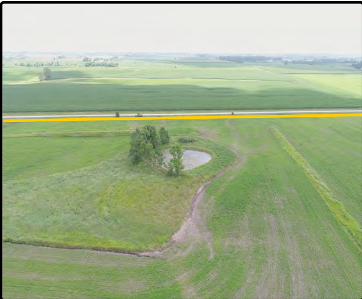
SE corner; retention pond
