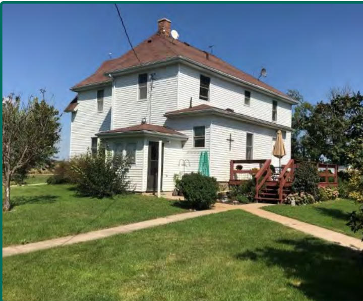
Southwest corner of house
