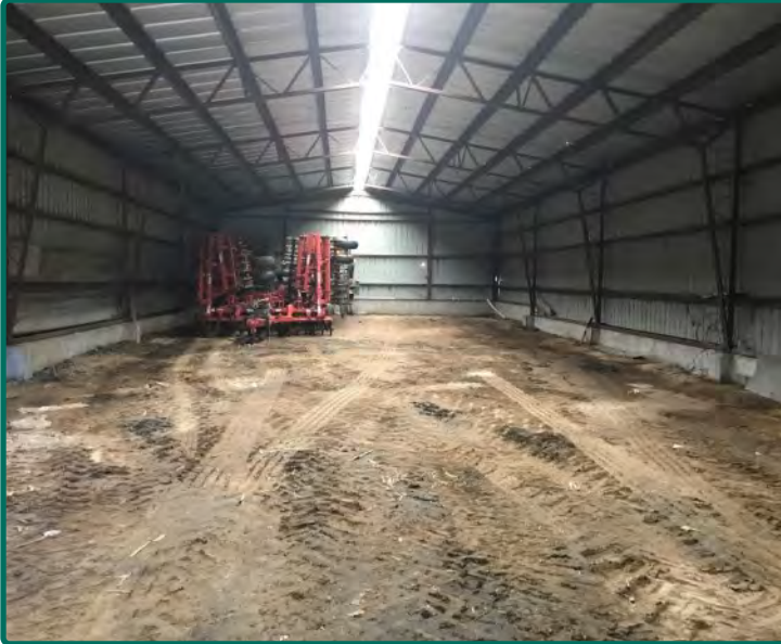
40' x 100' Utility building
