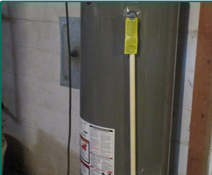
Water Heater Installed in 2014
