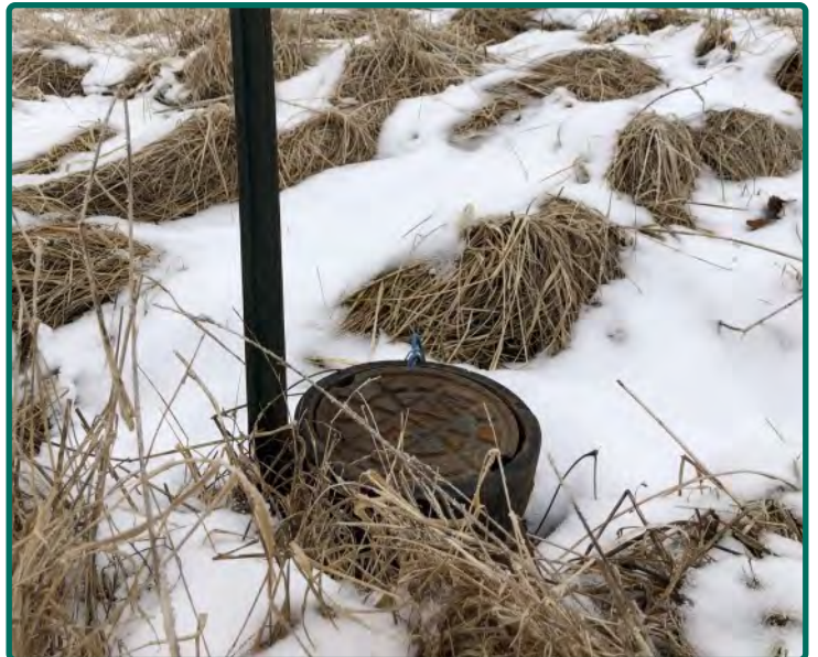
City water on south parcel and north parcel
