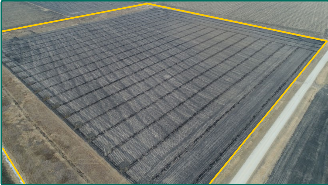
View from southeast corner on December 16, 2017 showing tile trenches
