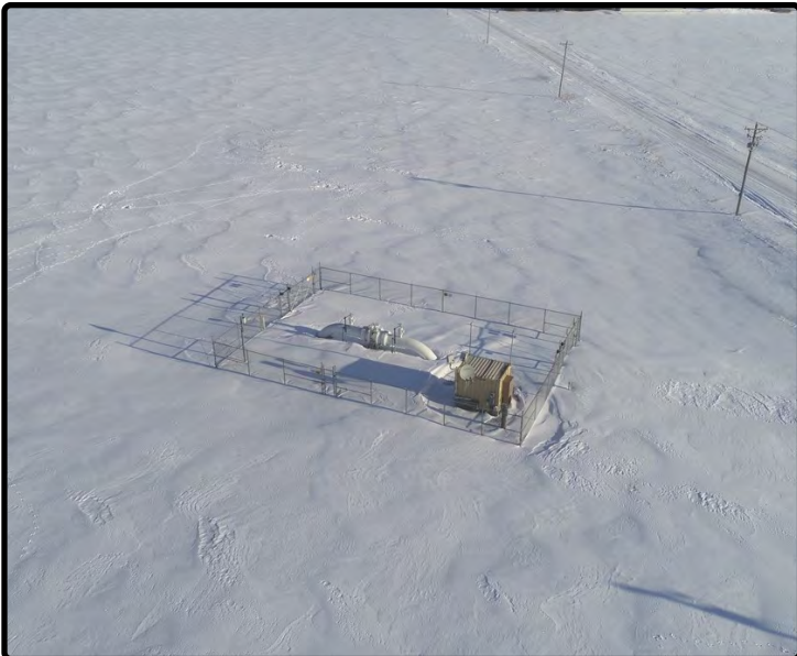
Pipeline Valve Site & Easement
