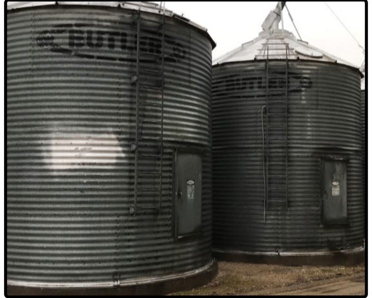
Feed Mill Grain Bins
