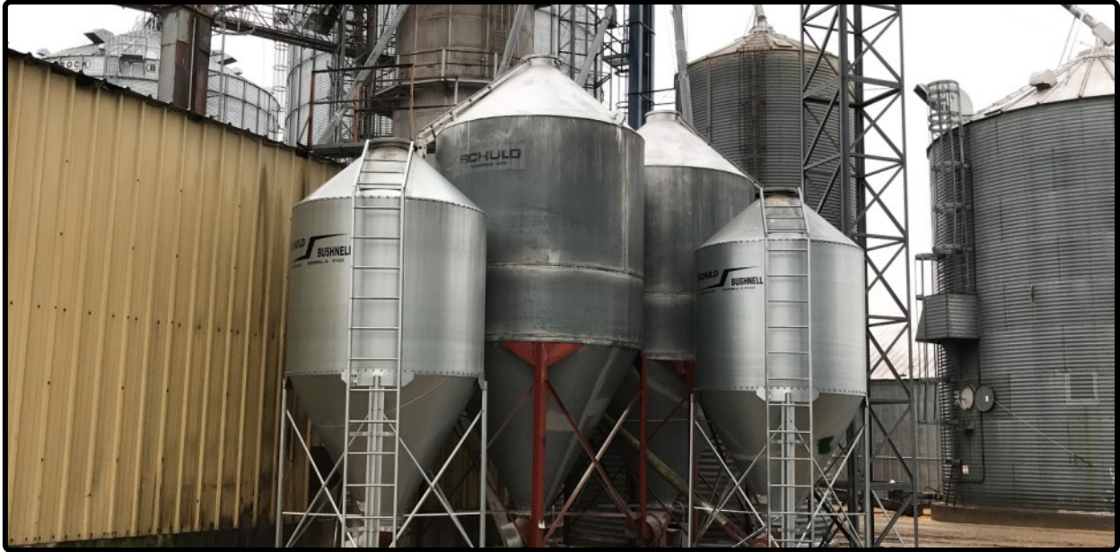
Feed Mill Bulk Bins
