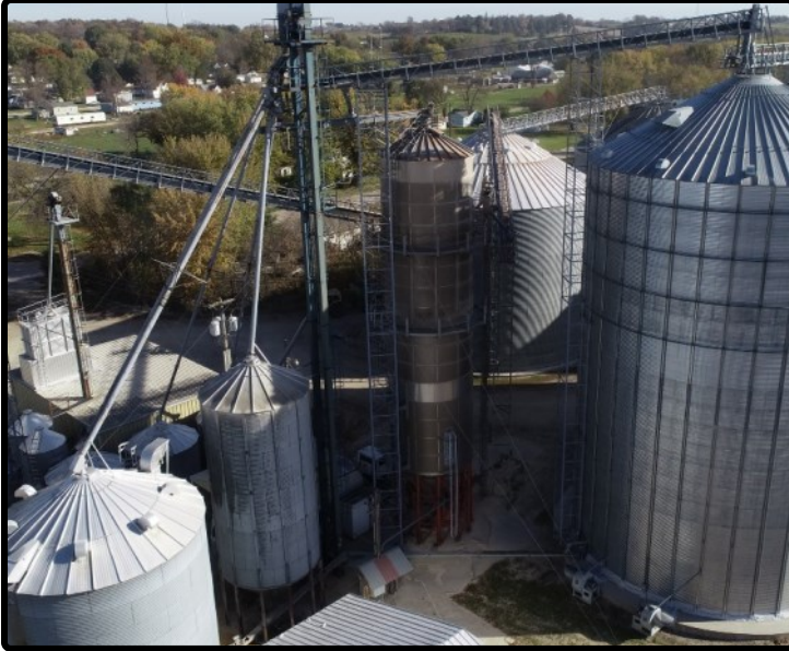
Grain Dryer & Bins
