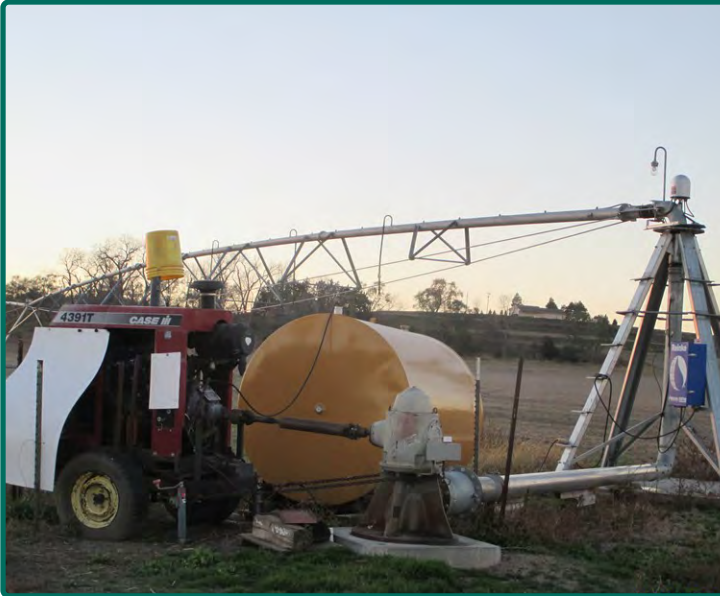
Pivot with Motor Well, & Diesel Tank
