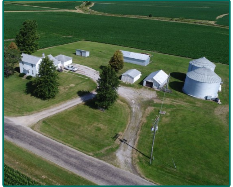
Section 6 - Building site
