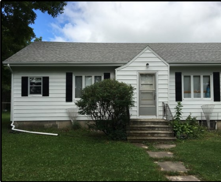
House-East Side (Front)
