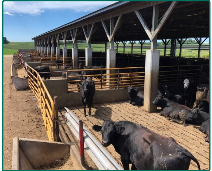
540-Head Cattle Facility
