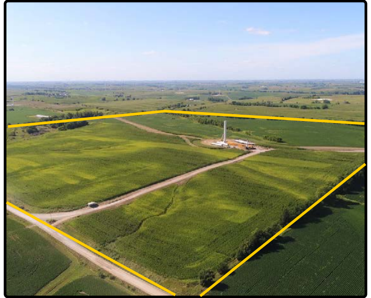
Southeast Looking Northwest
