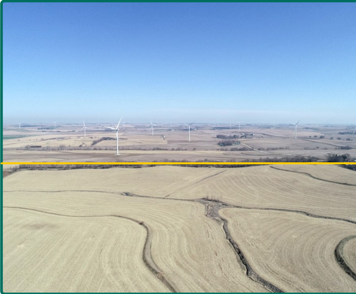
View from 230th St South
