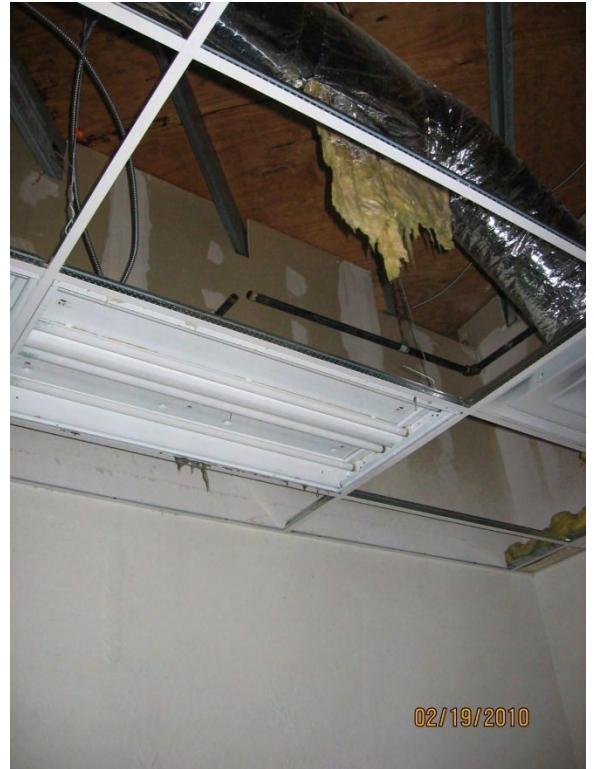
Photo 22 – Sprinkler system leak from February
