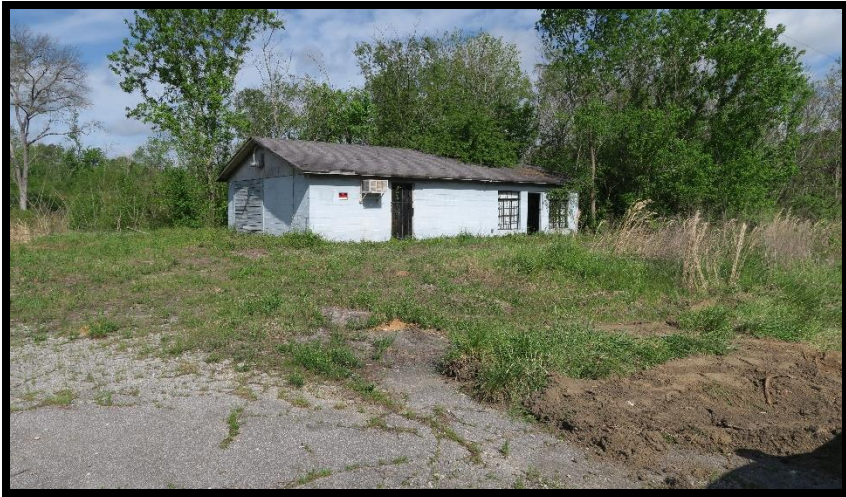
Building prior to demolition, taken September 25, 2017 (provided by Mr. Philip King)
