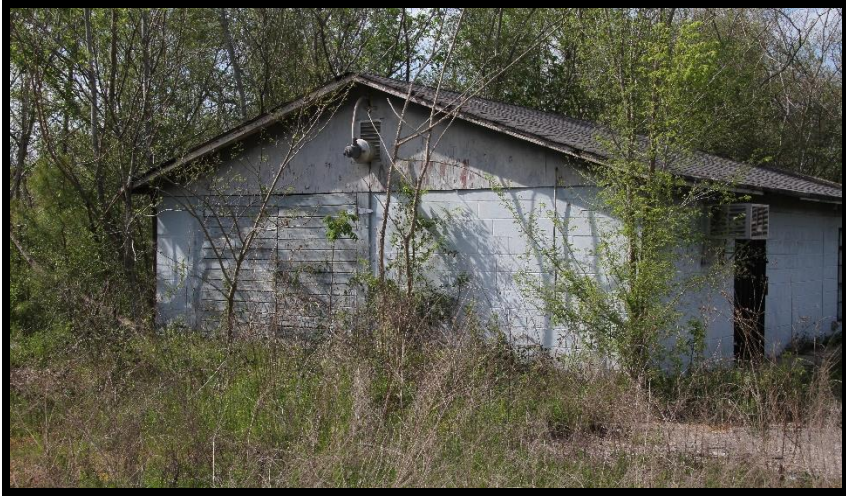
Building prior to demolition, taken April 11, 2017 (provided by Mr. Philip King)
