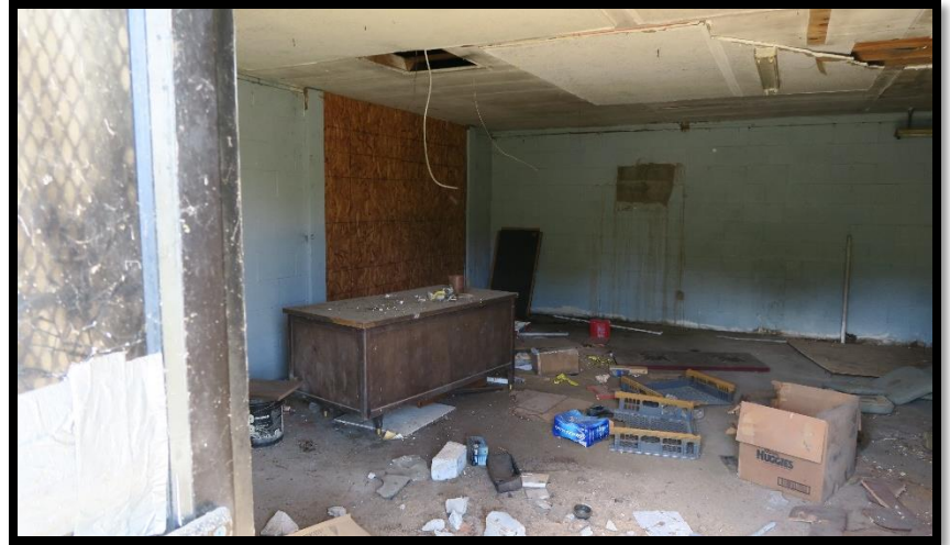
Inside of building prior to demolition, taken April 18, 2018 (provided by Mr. Philip King)
