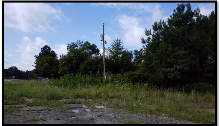
Pole mounted transformer (no signs of leaks)
